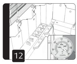
With all legs now connected, open the lock off valve and pressurise the brace against the trench sheets to approximately 1000psi, unless otherwise stated.
