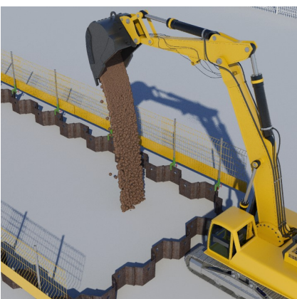
7. Reinstatement can then continue to ground level.
