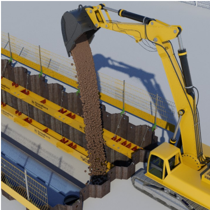
1. Backfill to the underside of the lower frame.
